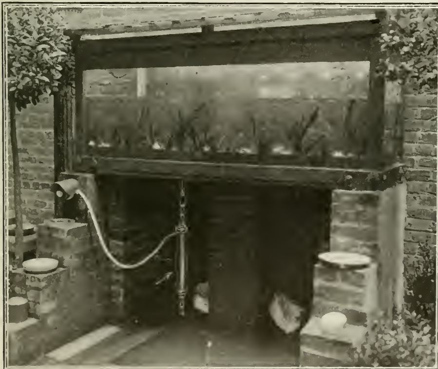
This Picture Shows How an Electrical Heater (See Arrow) Was Adapted to Warm the Water in a Fish Tank Containing Tropical Members of the Finny Tribe.
