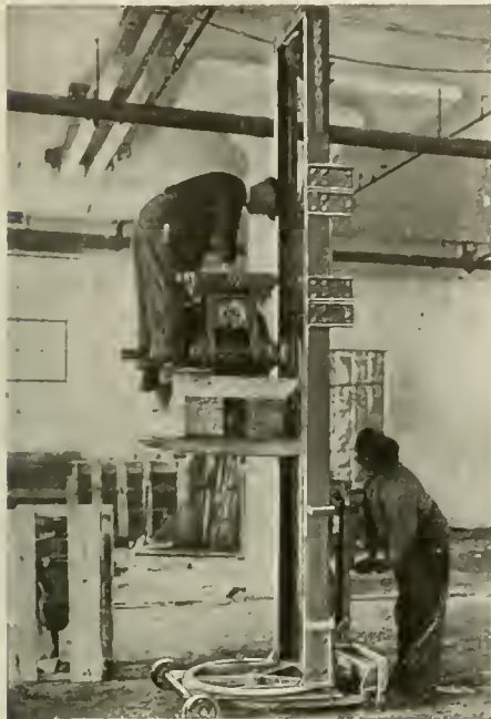
A Time and Labor Saver Which Every Electrician Will Appreciate, is This Latest Portable Elevator for Erecting Ceiling Motors.
