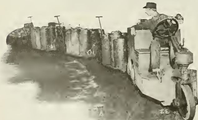
Fourteen of These Busy Electric Locomotives Haul Heavy Loads Up to 15 Miles Per Hour in One Industrial Plant. They Operate on Storage Batteries.
